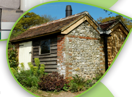
Grade 2 listed boiler house shed
